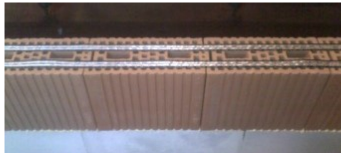
Figure 16 – Armature de joint horizontal
